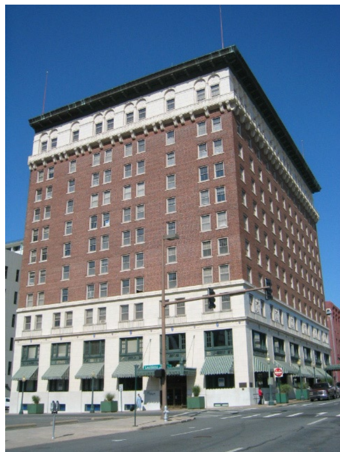
Figure 4-4. Medium density office space
