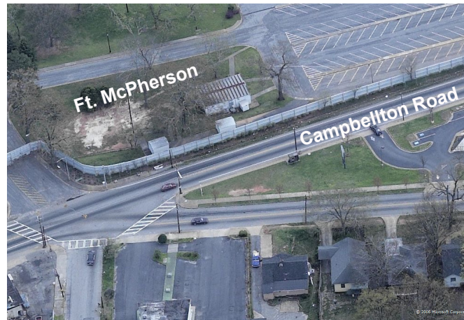
Figure 2-17. Campbellton Road along the northern boundary of the site
